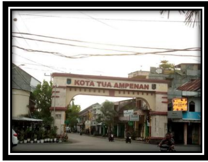
Figure 6. The entrance gate of Ampenan Old Town (Source: authors documentation, 2024)
