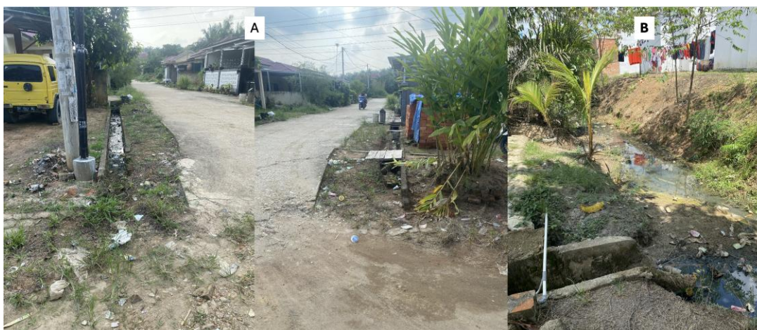
Figure 3. A. Disconnected household drainage system that flows onto the ground and concrete-paved road; B. Artificial canal functioning as the main wastewater drainage channel, but has become silted
